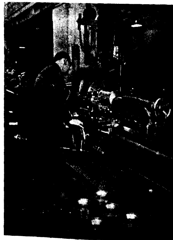
Fig. 3. Swift 8V3 Lathe turning cast iron sleeves at Taylor and Challen Ltd., Birmingham.
