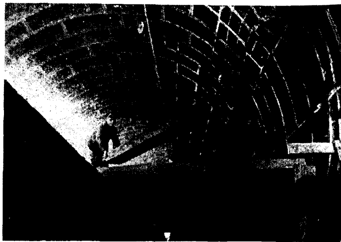
Construction of a passenger platform of the USSR Agricultural Exhibition Station of the Moscow Metro.
