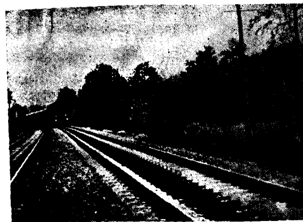
The modern French tracks are made up with rails 800 meters long. Fixed on the sleepers with elastic joints.
