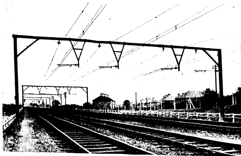
Four-track, broad flange beam portal structure. Showing a method of "registering" (i. e. locating) the contact wire and auxiliary catenary wire over each track. The wires are arranged in compound catenary form.—London to Shenfield Electrification.
