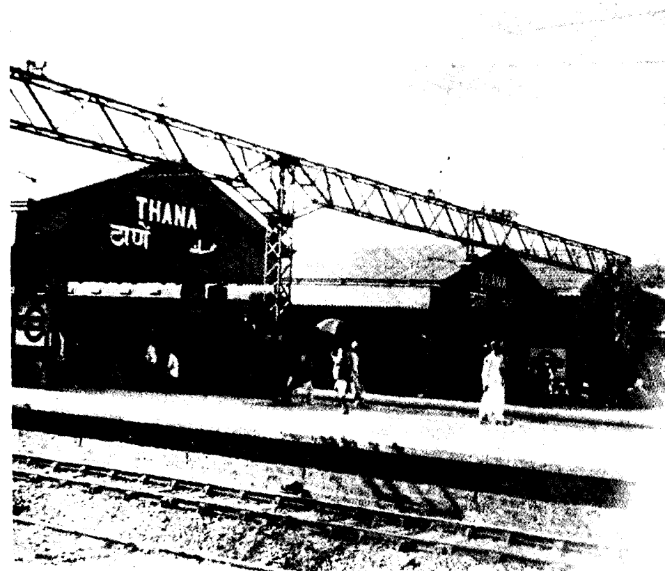
Lattice-type supporting structure at Thana, Central Railway, India. Note the bird guards over the insulators to prevent accidental earthing of the overhead equipment.
