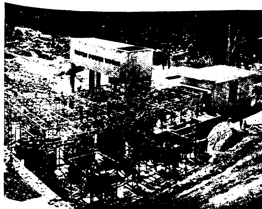
Sending end substation with power house in the background.
