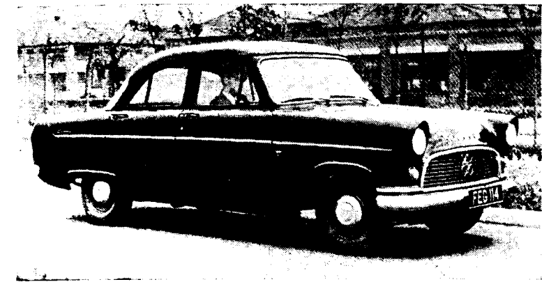
Ford Consul Car fitted with Perkins Four-99 diesel engine
