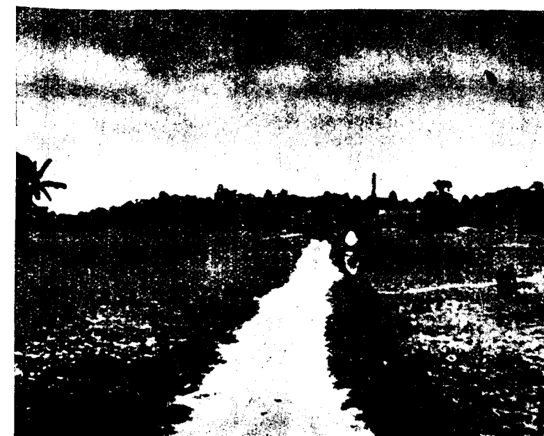
The fifteen-feet broad Keyapukur Road has thus taken shape with a height 5 to 8 feet. Inaccessible villages have thus been linked with the outside world by this enviable stretch of road as an artery of rural life.
