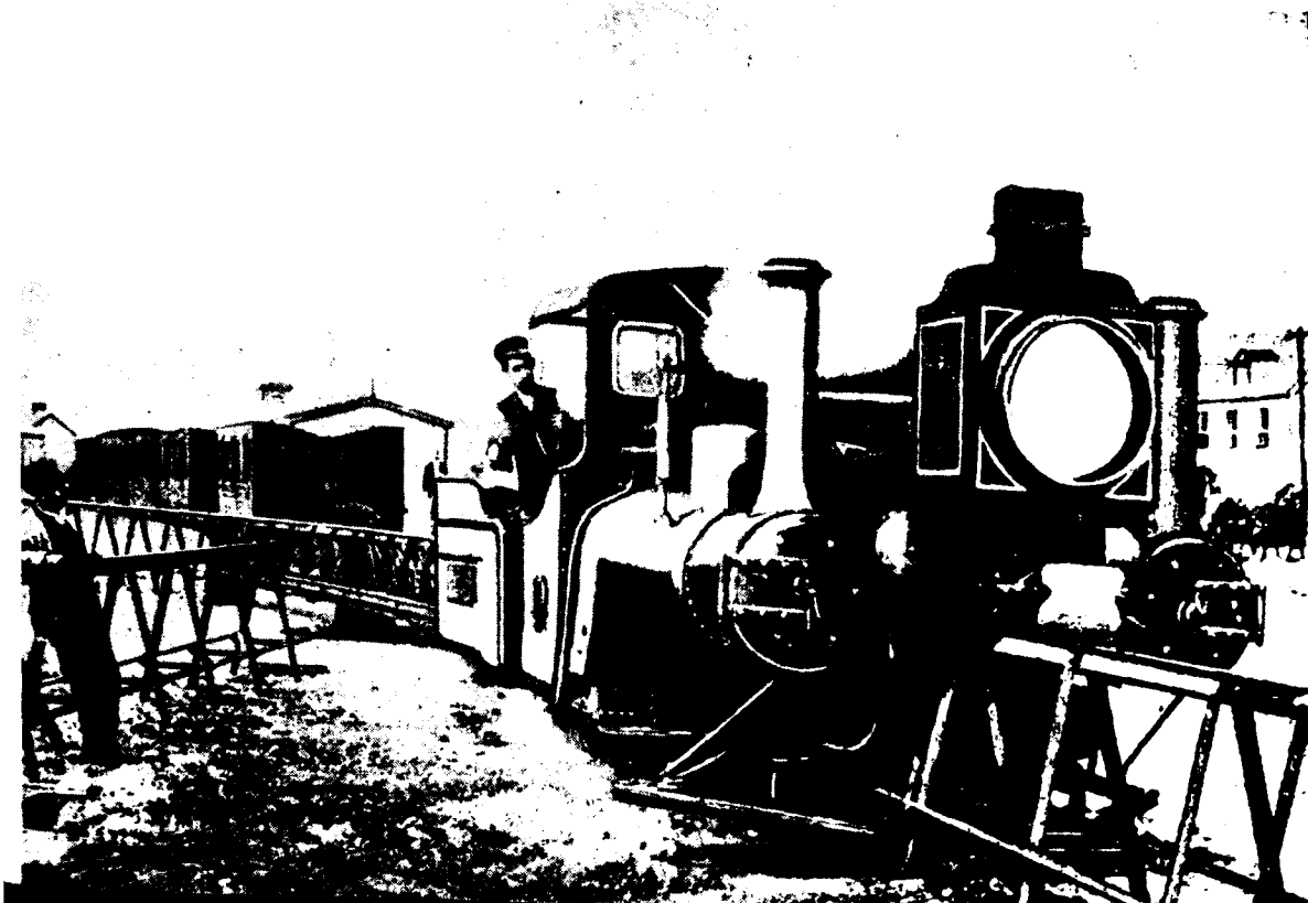
Listowel terminus of the Listowel and Ballybunion Railway, in the nineteen-twenties, showing the curious "Siamese Twin" Locomotive and divided passenger cars in rear
