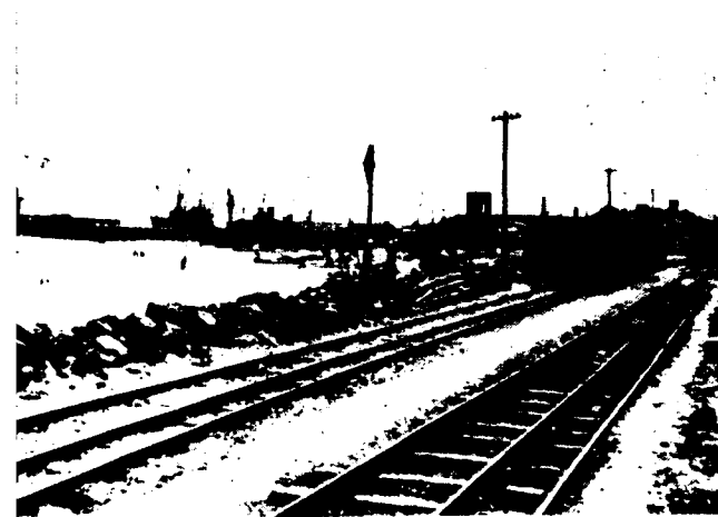
New tracks laid on the foreshore of Madras Harbour
