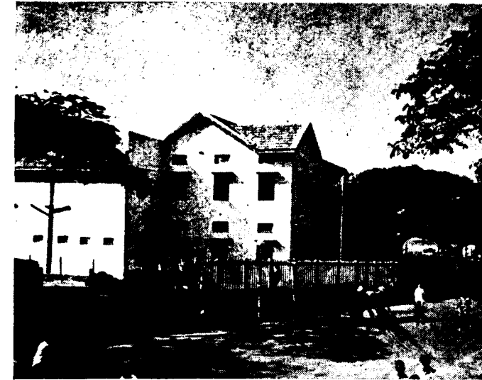
A view of the newly built Running "Room"
