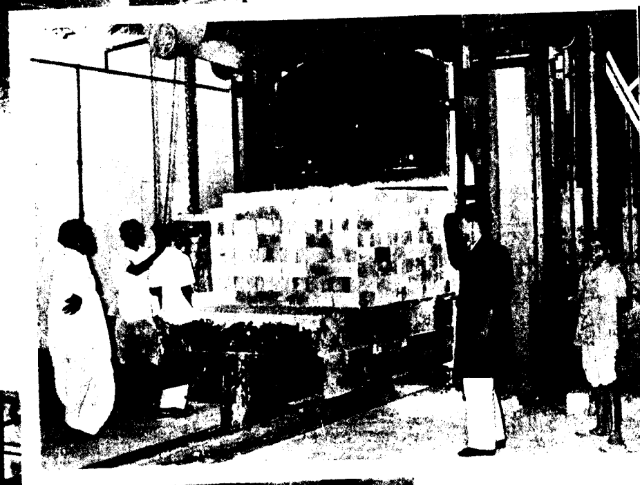
FIG. 5. — THE BRICKS LOADED IN A CAR ARE PUSHED INTO THE FURNACE FOR FIRING.
