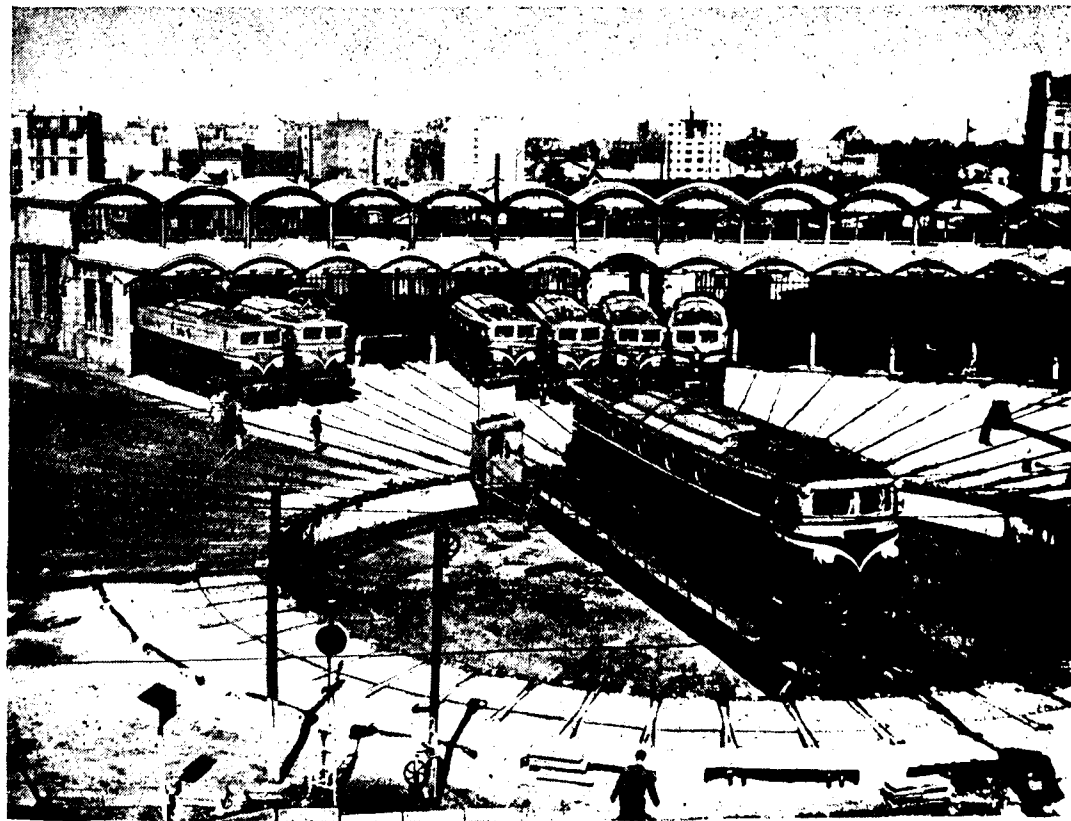
Depot for electric locomotives at Charolais (Paris-Lyon)
