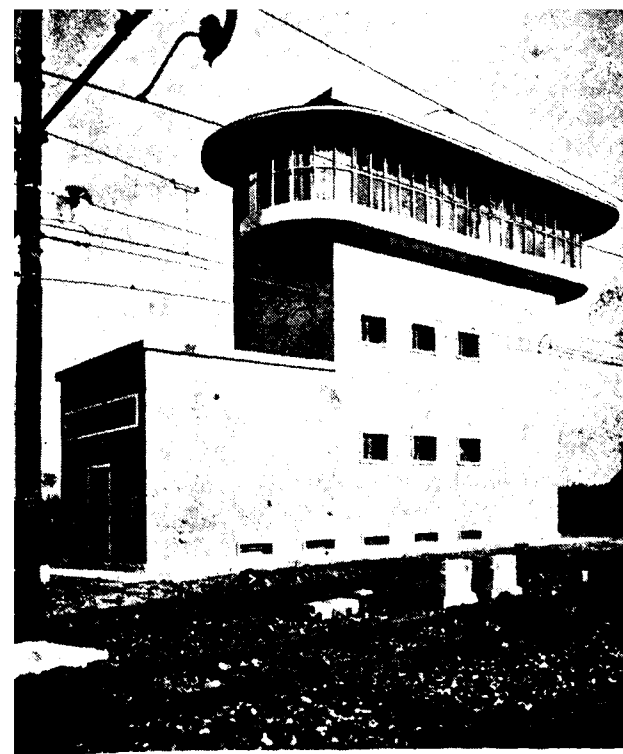
A typical modern signal box on the Italian Railways outside Naples
