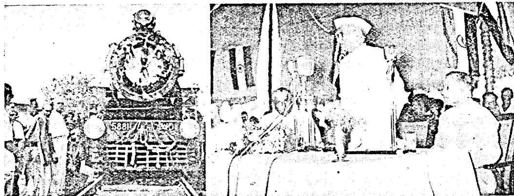
Opening of the Indore-Dewas-Ujjain Broad Gauge rail line. (Left) The first train steaming out. (Right) Dr. K. N. Katju inaugurating the line.
