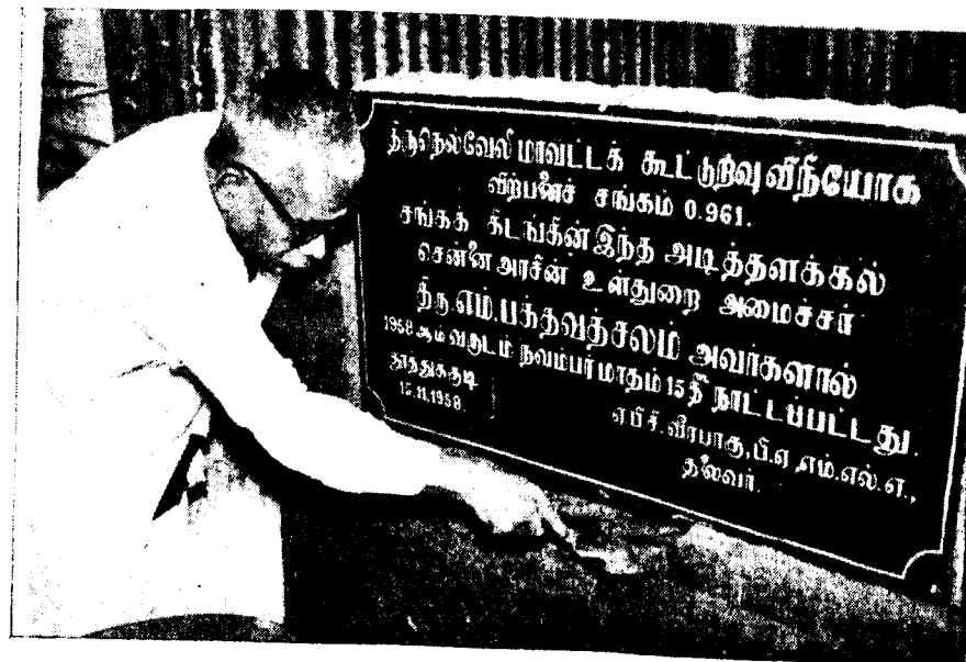
Sri M. Bhakthavatsalam, Home Minister is seen laying the Foundation Stone of the Godown.
