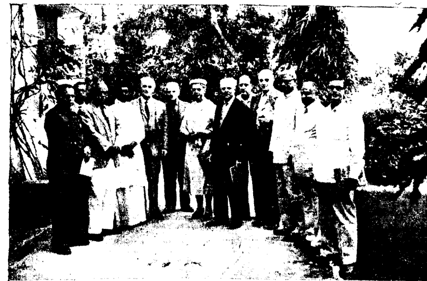
The Members of the I.C.A. Delegation inspected one of the houses constructed by the Co-operative House Construction Society at Madras. Sri Rathnasabapathy, President of the Society took them round the Colony.
