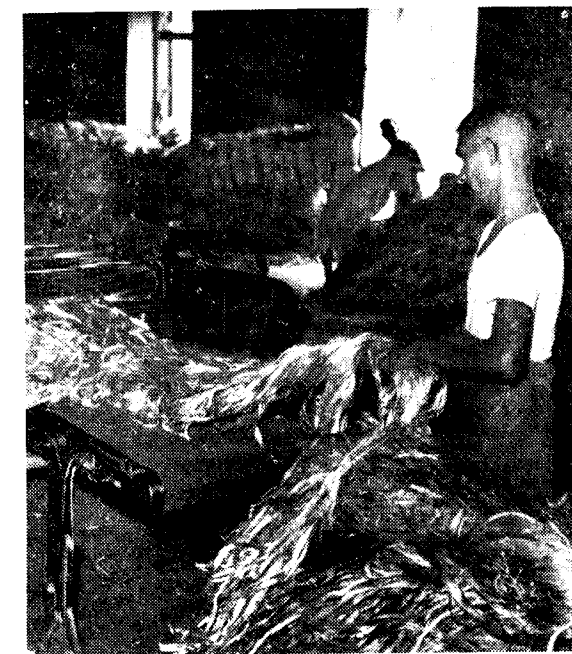
Jute being delivered from a softener machine
