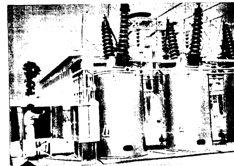
The Sarda Power House has an installed capacity of 41,400 KW and is the largest hydro-electric station in Uttar Pradesh. The English Electric Company supplied, erected and commissioned all the plant for this Power House. Above is shown one of six 'English Electric' 132 kV Oil Circuit Breakers installed at this site.
