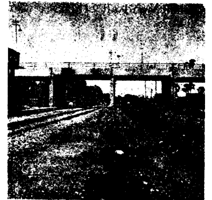
Photo 7. Overbridge at Patna over Eastern Railway Main lines.
