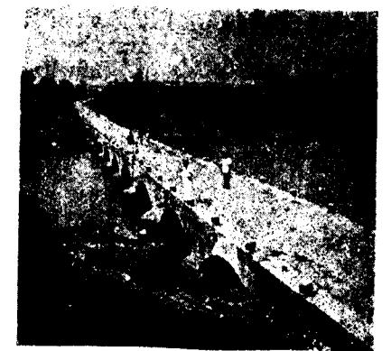
Photo 10. The Sanjoy submersible bridge.
