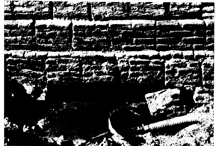
Photo 3. Condition of masonry of the Plate Girder Bridge.
