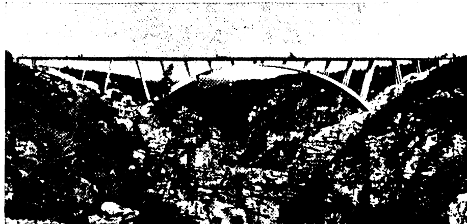
Photo 1. The Storms River Bridge, South Africa.
