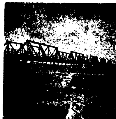
Photo 5. The Gumani bridge.
