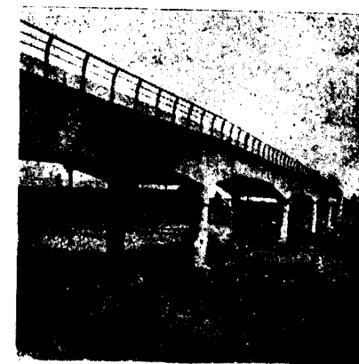
Photo 9. The Kitchinia bridge on Patna-Ranchi road.
