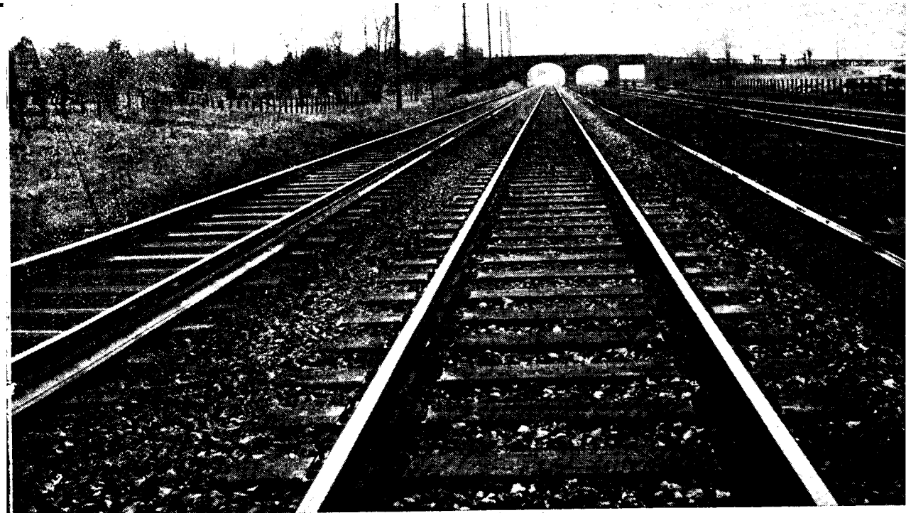
New standard flat-bottomed rails on the main-line of the Western Region of British Railways near Langley
