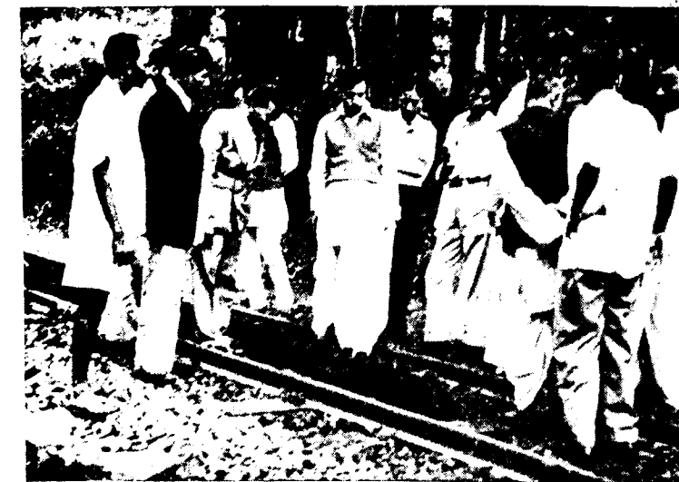
Inspecting Rack-Rail at Kallar
