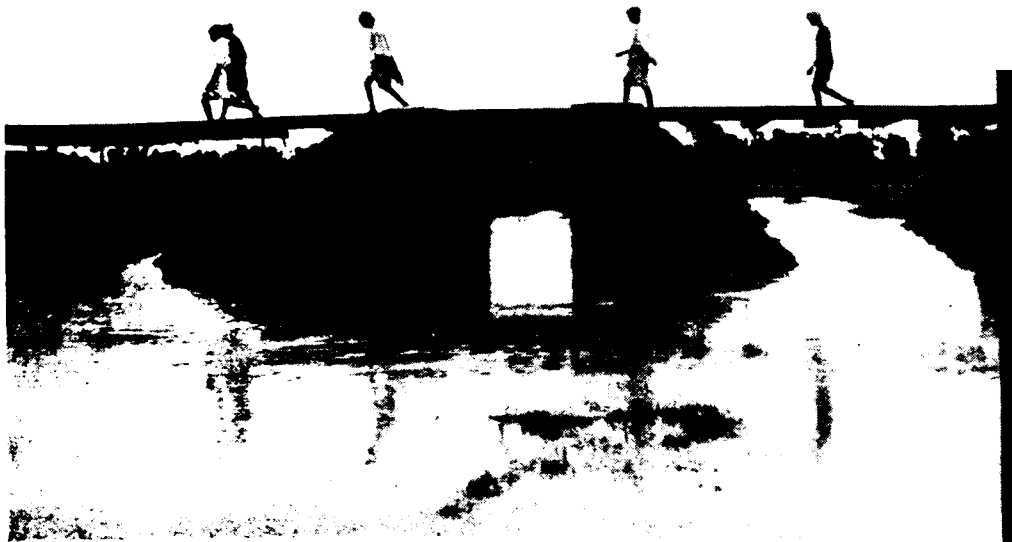
The bridge at the outer signal of Nayudupet Station with the embankments on either completely washed away by flood waters. The damage to this bridge was similar to that which occurred at Ariyalur
