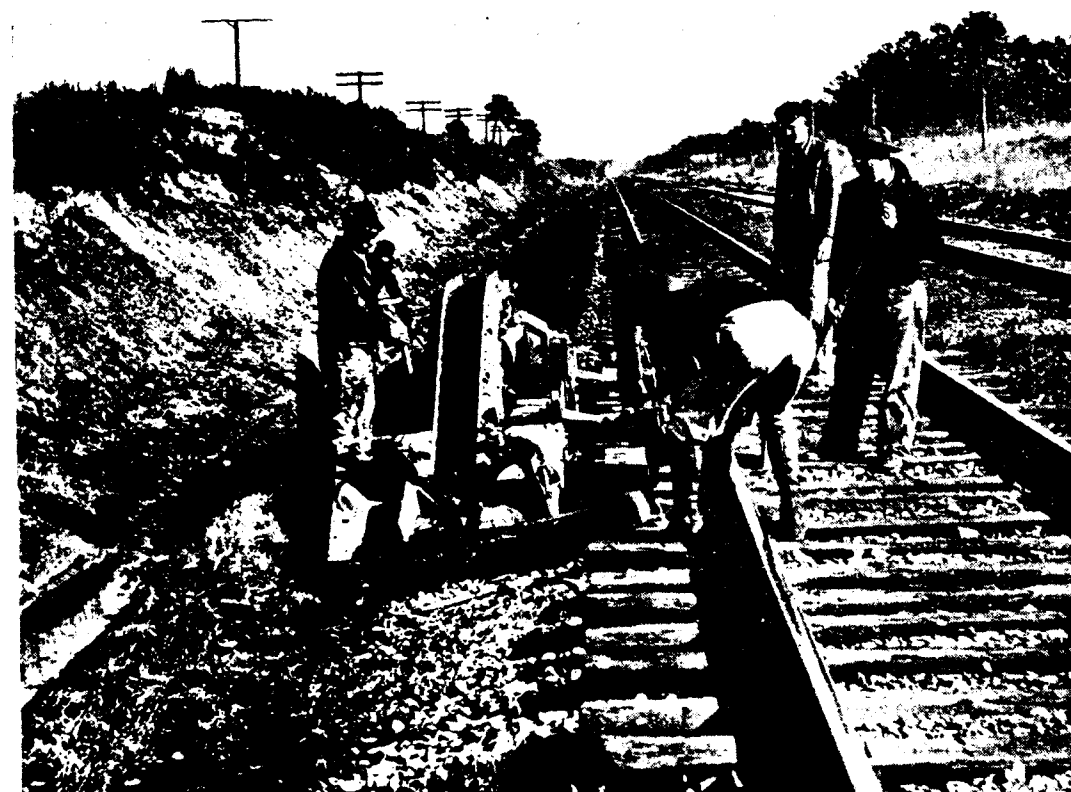
Ballast cleaning machine in operation on the ACL
