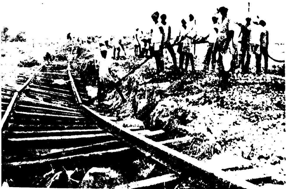
Railway Track washed off the bank near Dhoravani Chatram
