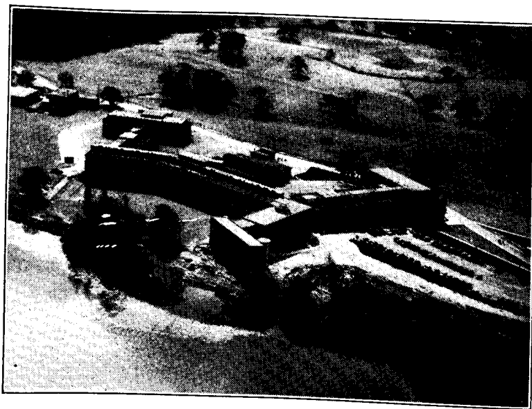
FIG. 1.—Aerial view of north aspect of the central laboratory block, showing Radnor Mere in the foreground and the general appearance of the surrounding parkland. The separate building on the left of the picture is the boiler house and workshop, and the trees behind it screen from view the building for the animal breeding unit.
