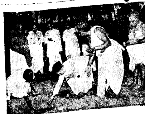
Laying of foundation to the S.I.T.U. Building
