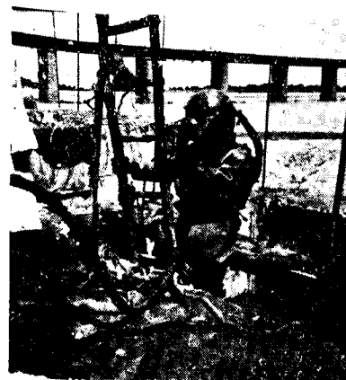
Photo 1. Reinforcement for well kerb 6" x 6" x 1/2". angle iron can be seen at bottom
