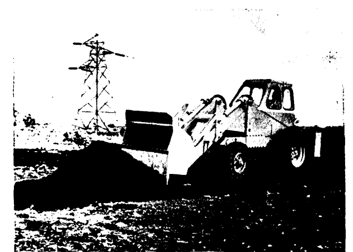
Fig. 3. Levelling refuse in controlled tipping with the bulldozer blade attachment.
