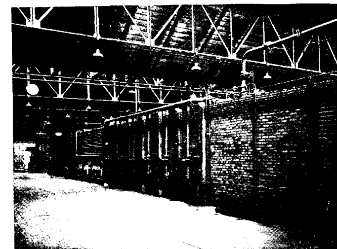
Fig. 7. Tunnel kiln—firing zone.
