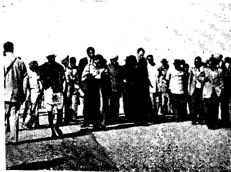
Delegates inspecting surface treated stabilised soil roads near Batala (Punjab)
