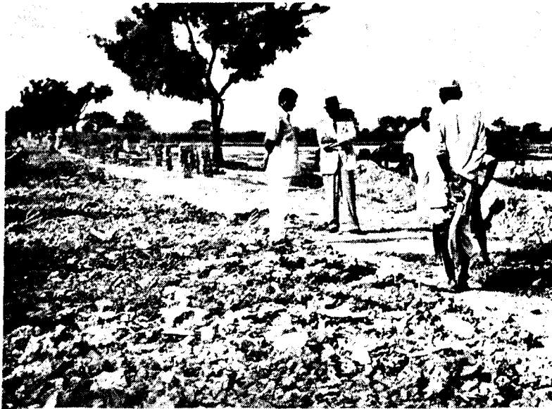
Photo 4. Delhi-Meerut Road. Excessive deformation leading to failure of road which is dug out and is being relaid.
