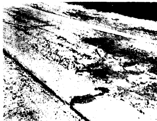
Photo 2. A close view of C.C. pavement of G. T. Road showing settle- ment and disintegration of C.C. slabs
