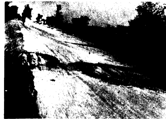
Photo 9. Meerut-Baghpat Road - A closer view of the road in mile 7, fig. 6 that has failed showing com- plete disintegro- tion of the crust. The pulpy earth from beneath has come up under the wheel pressure
