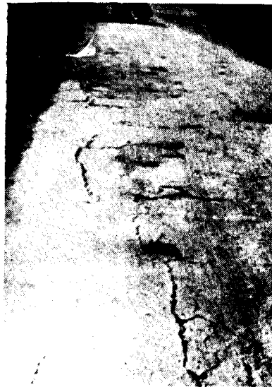
Photo 5. Meerut-Baghpat Road showing initial stage of the road surface breaking
