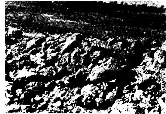
Photo 7. Meerut-Baghpat Road showing heaps of earth taken out from below the road surface which has failed
