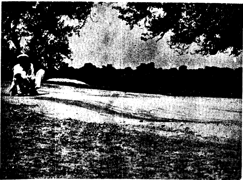
Photo 1. Muzaffarnagar-Shamli Road, mile 9/1 showing excessive deformation
