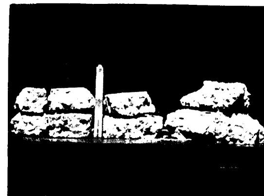
Photo 3. Showing concrete blocks taken out of C.C. slabs from G. T. Road for investi- gation (Note the varying thickness of slab 6 in.-4 in -6 in.)
