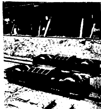
Photo 15. Locally built trollies for conveying beams
