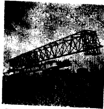
Photo 34. Launching girder moving over girders already laid in position
