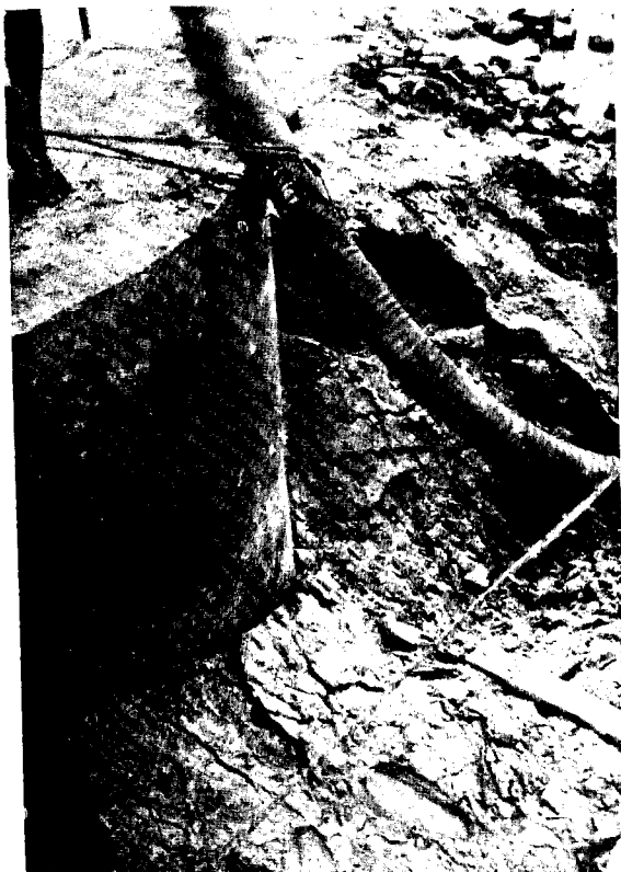
Photo 3. Subsidence outside the well when a sand blow occurred.
