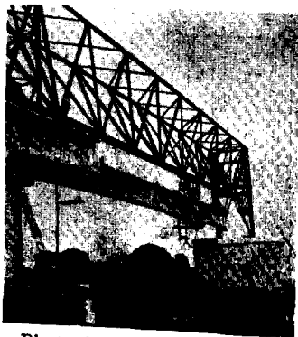
Photo 37. A beam being launched by the crabs and transport car II
