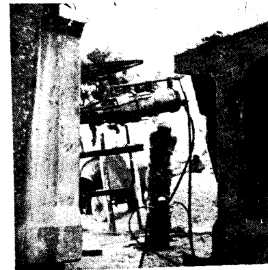
Photo 7. Prestressing in progress
