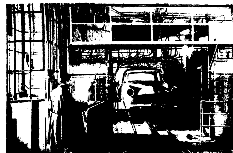
The body of a new "Volga" passenger car being painted in the electrostatic Chamber at the Molotov Automobile Plant in Gorky.
