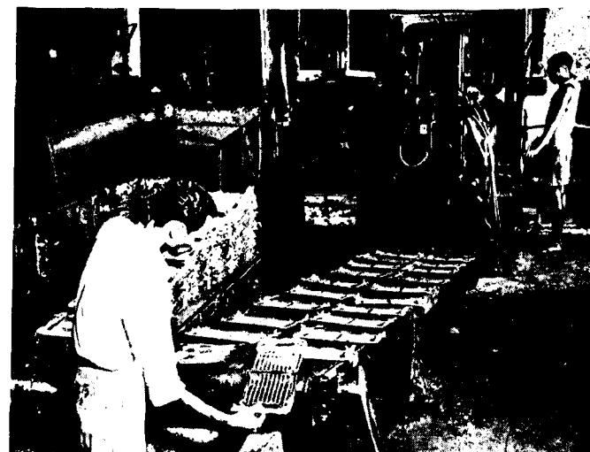
Automatic casting of plate-grids
