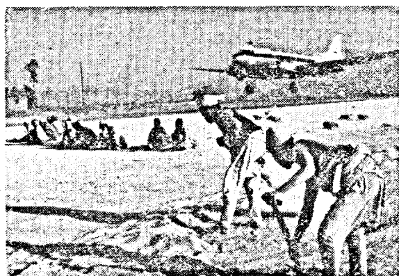
Building a permanent air-strip at Gaucher
