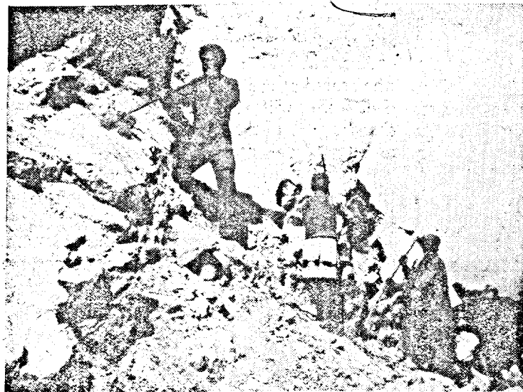
Army Engineers dynamiting granite rock for the construction of Tribhuvan Rajpath, the first
