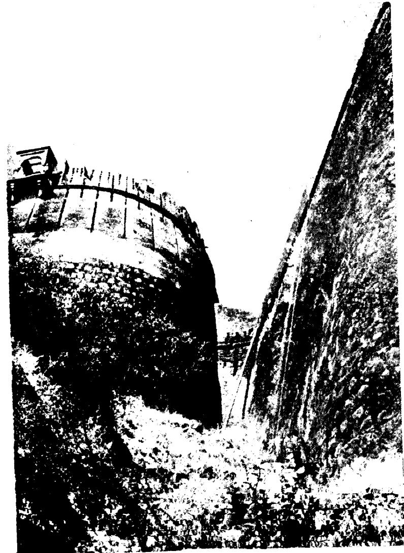
Picture shows the part of the fort from where burglars made an entry into the Maheshwar temple. The pole used by them to climb the wall may also be seen.
