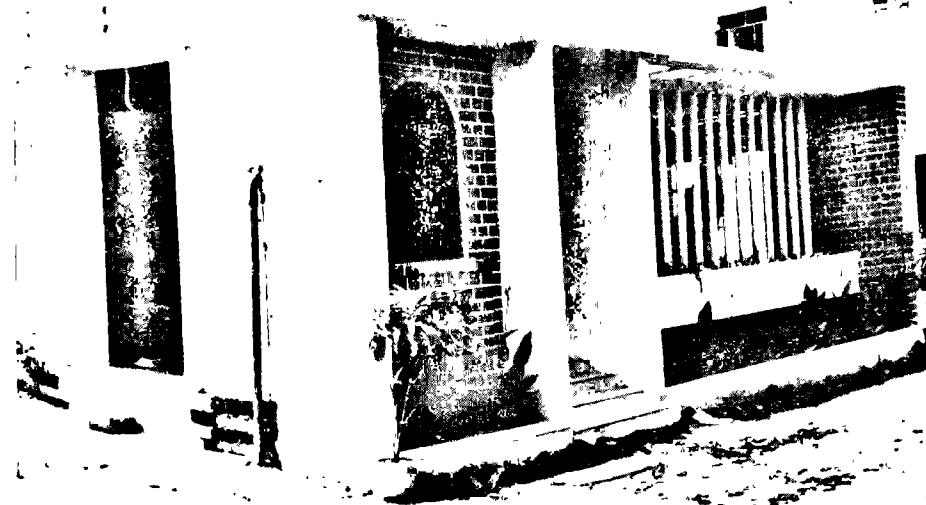
The 18" thick concrete walled building specially designed to house powerful radio active machine.
