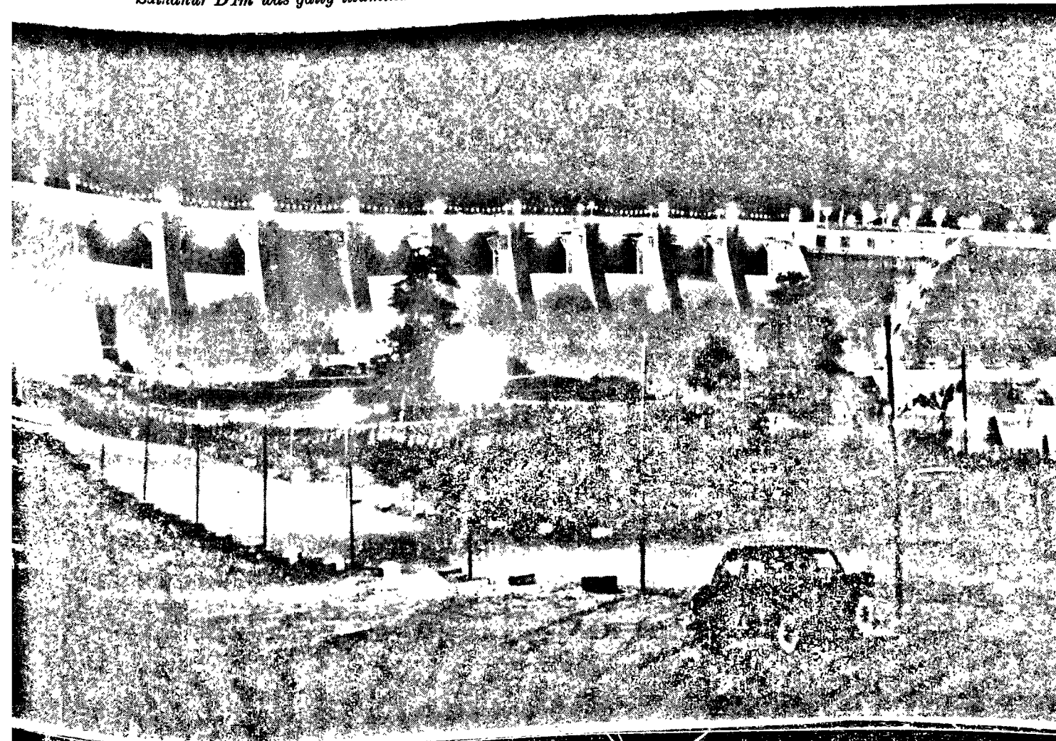
Sathanur Dam was gaily illuminated on November 10, 1957, when waters were let out for irrigation.
