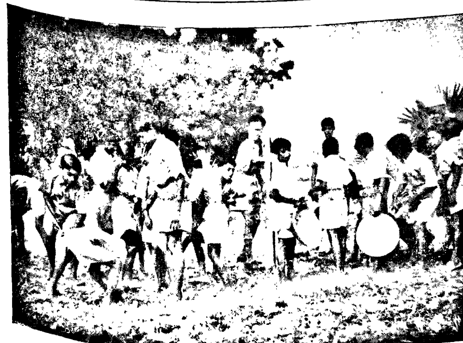
Block Development staff of Maduranth gam contributed Shramdhan with the villagers to lay an earthen road at Mudukarai village during last month.
