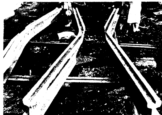
Fig. 11. Welding preparations at a mounting tongue consisting of heavy web rails
