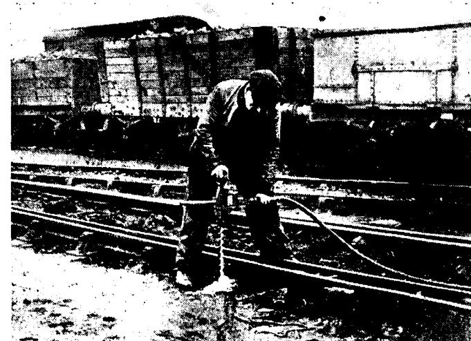
Drilling holes for Chair Screws with an Armstrong Whitworth Woodborer Size 362 RHW.
