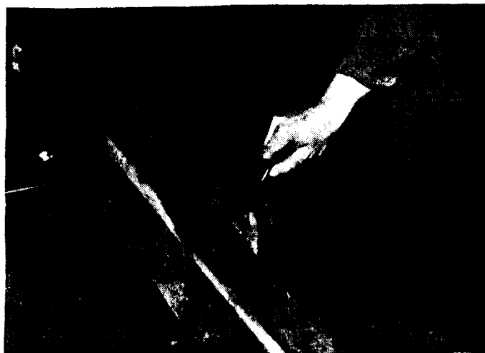
Fig. 15. Repairing the point of a tongue by the autogenous built-up welding
