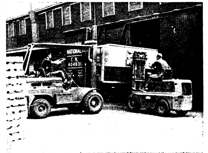
YL-4-1425—Two Clark Yardlift-40 unload plywood to a position where one may handle it from box car at Coutu Lumber Co., West Warwick, Rhode Island.
