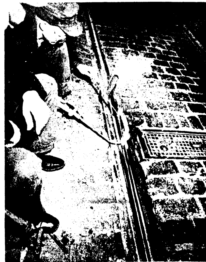
Fig. 17. Repairing a switch tongue by built-up welding on a rail in operation
