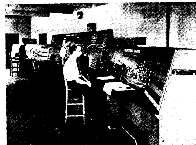
Fig. 6. Route relay interlocking control panels at Liverpool Street Station signal box.
