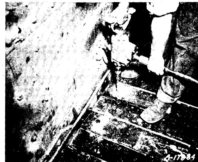
Drilling planks to match existing bolt holes.
