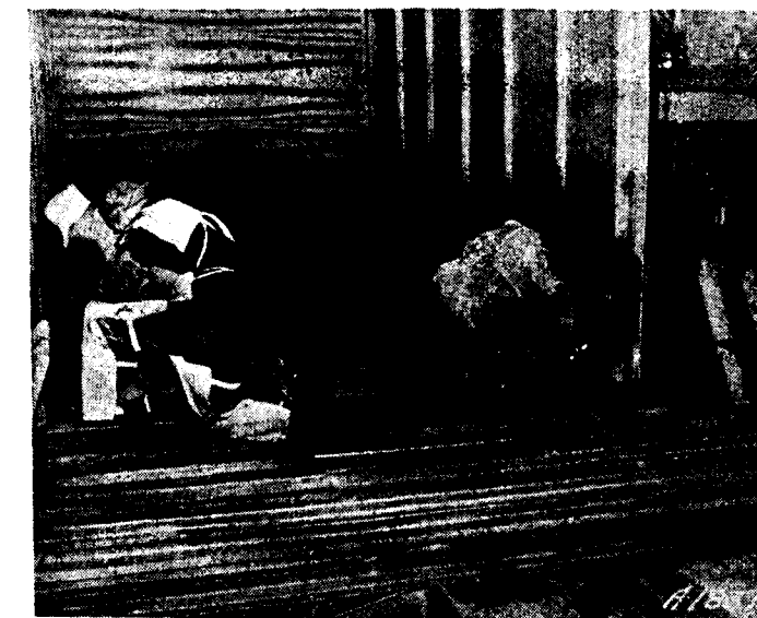
In this new box car installation steel ribs are being centered before welding to provide sealing space at car sides.
