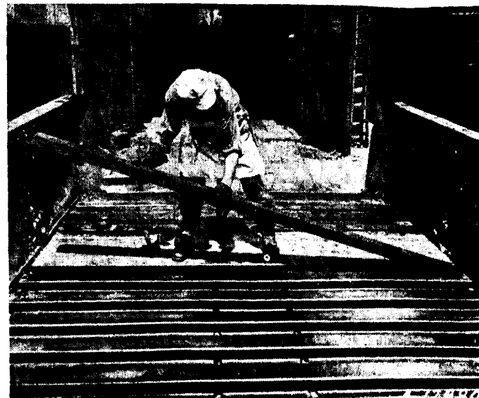
Laying treated wood planks between spray-painted ribs.
