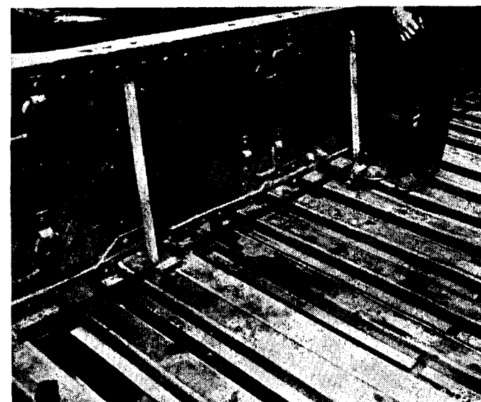
Spacing ribs with template. The one shown is half the length of the car, of welded construction and made to clear special ribs over bolster.
