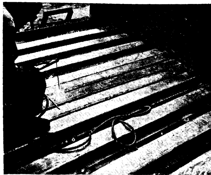
Welding special ribs over bolster.
