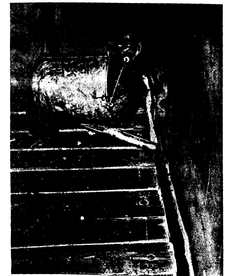
Pouring car cement after inserting galvanized closure strip and filling crevice with sawdust.
