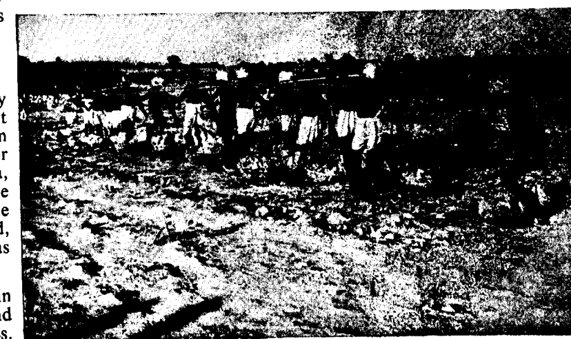
Levelling factory site : a procession of men workers balancing loads on their shoulders.
