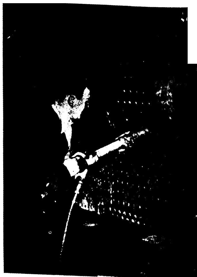
Removing Stay Bolt rivets from Loco. Fire Box with Armstrong Whitworth Size 9300 Rivet Buster.
