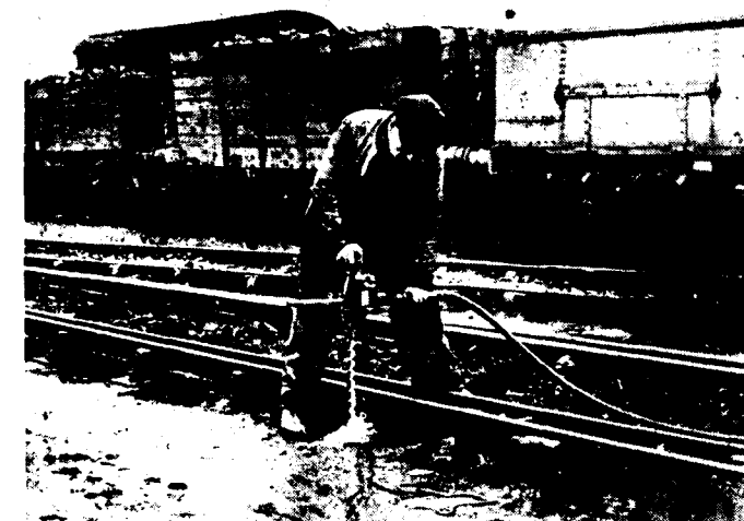
Drilling holes for Chair Screws with an Armstrong Whitworth Woodborer Size 362 RHW.
