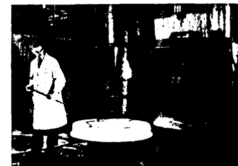
Fig. 20. Gauging Wheel after Dishing.
