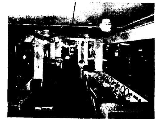
Fig. 14. Main Control Room.
