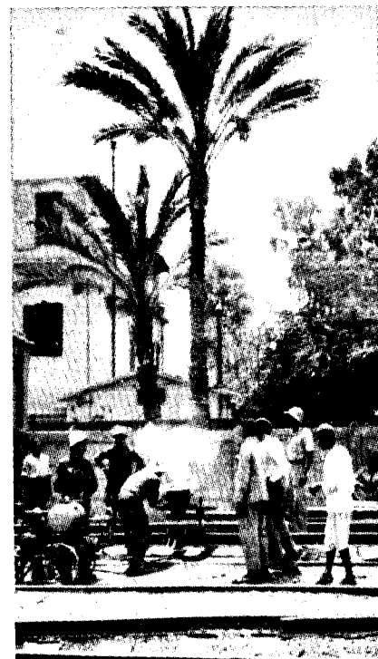
Welding in tracks.
