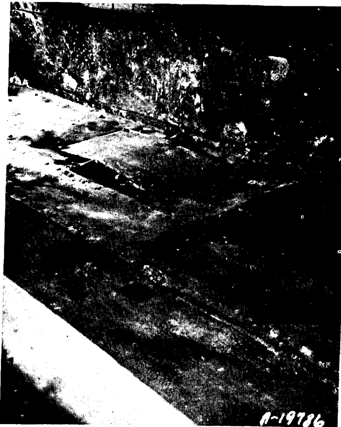
Steel plate floors become belled, perforated and unsuitable for even bulk loads.
