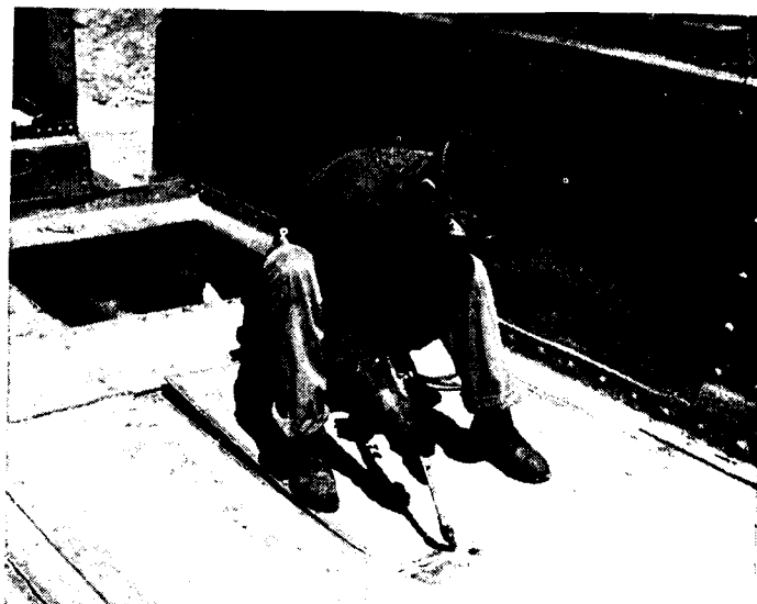
Stripping gondola car floor by cutting out old plate between sills and crossbearers in order to install the stringers. It is unnecessary to remove bolster or center sill cover plate.
