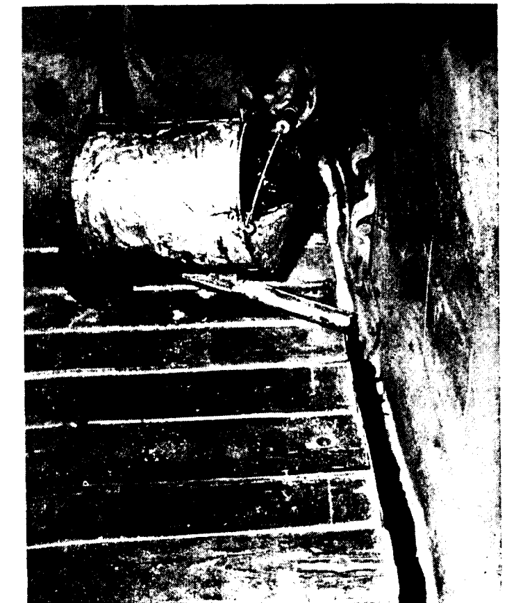
Pouring car cement after inserting galvanized closure strip and filling crevice with sawdust.
