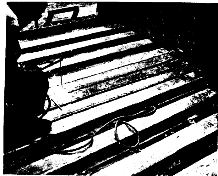
Welding special ribs over bolster.
