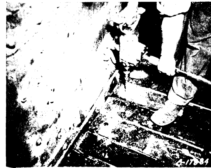
Drilling planks to match existing bolt holes.
