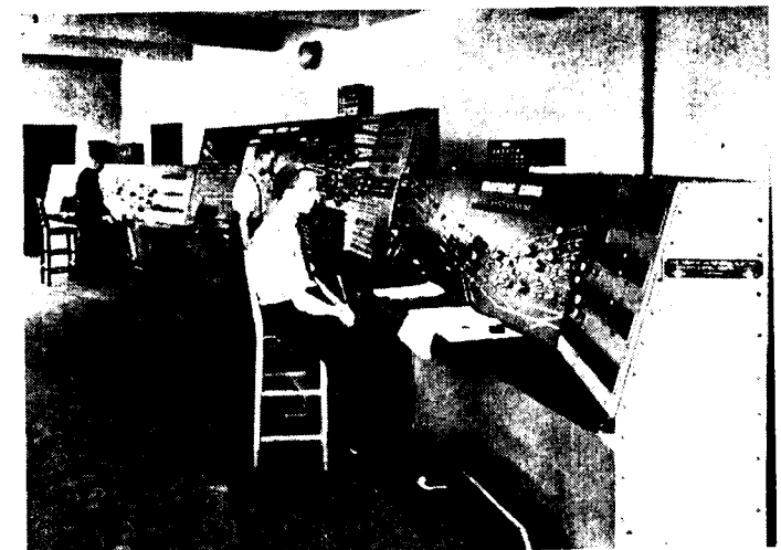
Fig. 6. Route relay interlocking control panels at Liverpool Street Station signal box.
