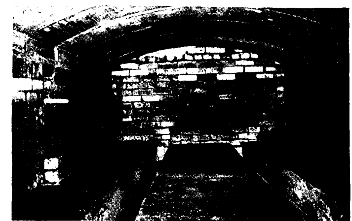
Fig. 7. Precast refractory concrete arch units and insulating concrete hearth of pit arch recovery furnace.
