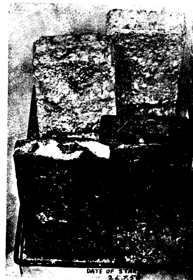
Fig. 8. Photographs showing condition of the brick-tile after about 3½ years of their partially embedding in soil containing 5 per cent sodium sulphate when viewed from different angles. The other deeply tar, impregnated brick-tile showed cracking of the upper top end.
