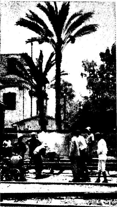
Welding in tracks.
