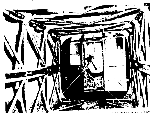
2. Subject seated in the cabin of the man-carrying centrifuge. A recording system picks up minute electrical impulses which are transmitted via the arm to the control room. These record changes in the subject's physiological condition. (Air Ministry Photograph, Crown Copyright Reserved)
