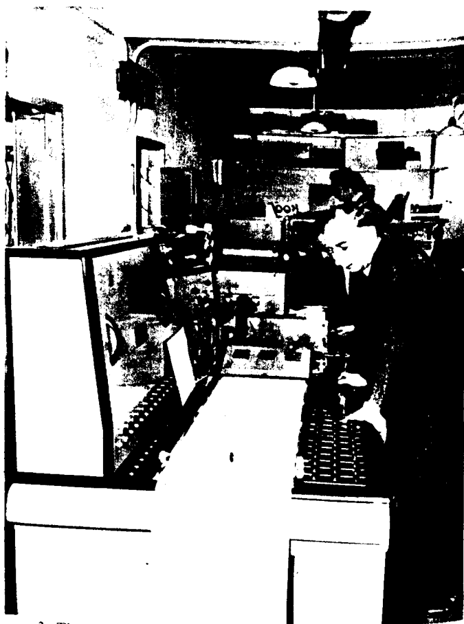
3. The control room showing (centre) the apparatus on which the changes in the physiological condition of the subject in the rotating cabin are recorded. ( Air Ministry Photograph, Crown Copyright Reserved )
