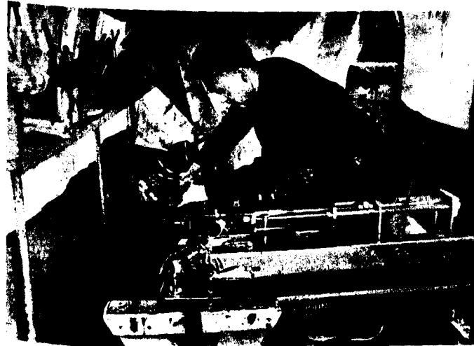
16. Taking a joint out of a mould during the construction of the Newfoundland link. (Courtesy of H.M. Postmaster-General)
