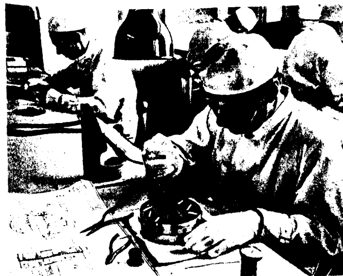
12. Wiring up directional filters for the rigid repeaters in the Clarendonville-Sydney Mines section of the system. (Courtesy of H.M. Postmaster-General)
