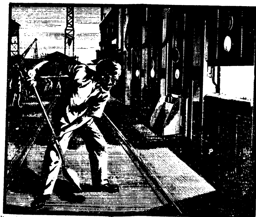
Shovelling dolomite into a recently completed 200-ton furnace in the new Steel Melting Shop.
