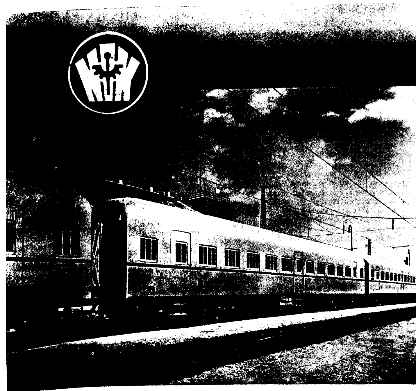
These third-class passenger coaches have been built for the Egyptian Republic Railways. Each accommodates 104 passengers, and features an extra door in the middle to facilitate the exchange of passengers at the stations.
