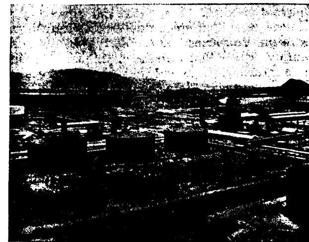
Fluid Cat-Cracker Unit feed tanks
