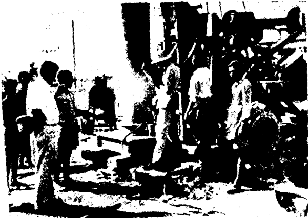
Welder at work—lowering casing in pumpwell
