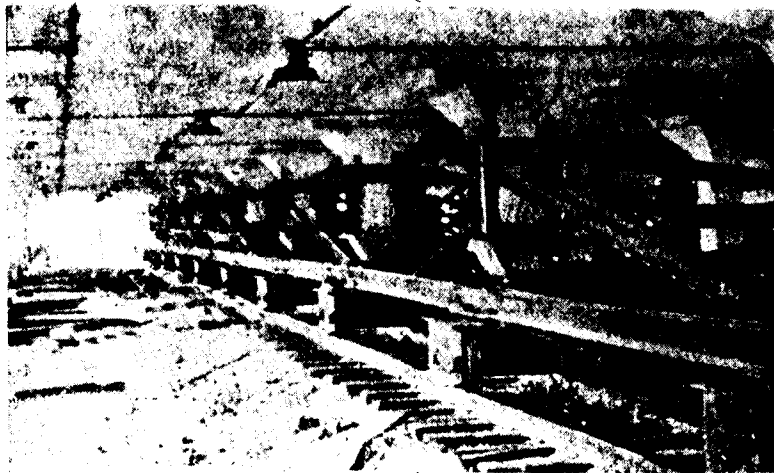
Fig. 2.—Underside of Building During Removal.
