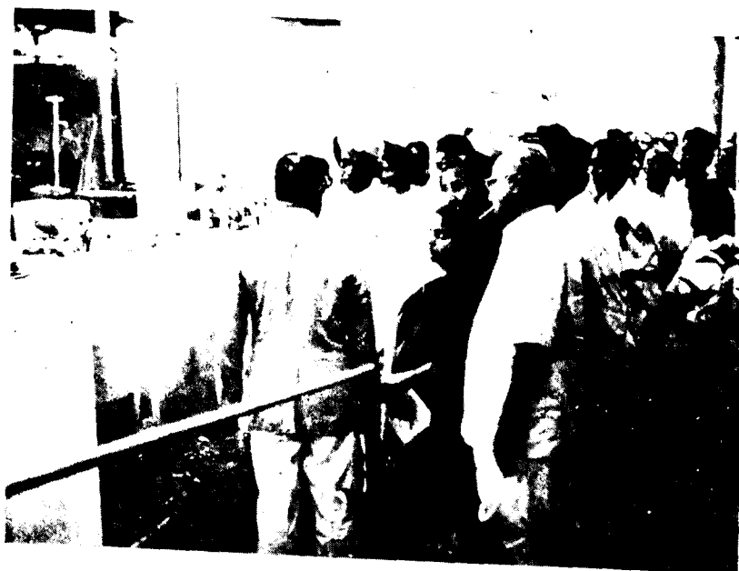
The Exhibition was opened by Sri C. D. Deshmukh, Sri K. K. Nambiar, Chief Engineer is explaining the model of a bridge construction to the distinguished visitors
