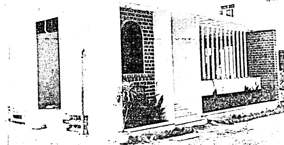
The 18" thick concrete walled building specially designed to house powerful radio active machine
