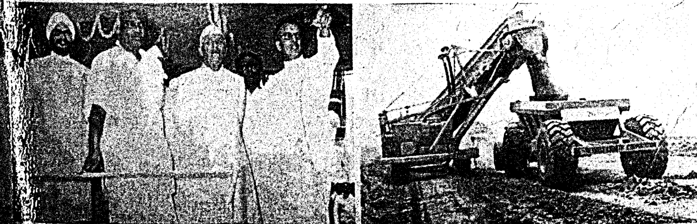
Giant earth-moving machines have started cutting the mine-face at Neyveli. These scraper loaders can cut and load earth at 900 cubic yards per hour.
