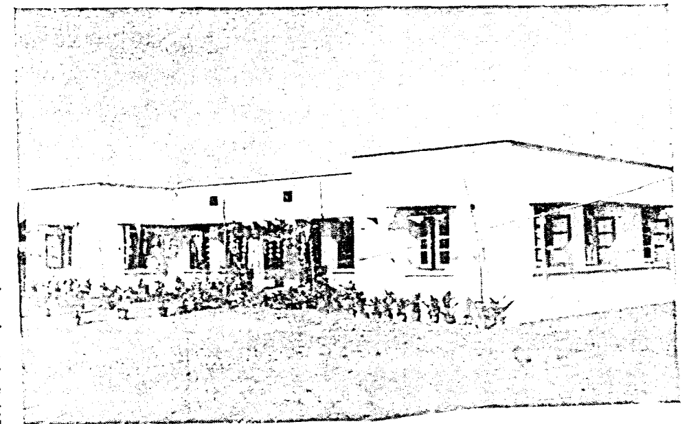
Children's Dormitory in Shaligram Boys Home donated through the good offices of the Victoria Branch of the Save the Children's Fund, Melbourne.
