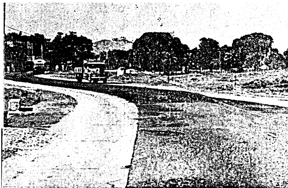
A conphalt road for high speed and heavy traffic.
